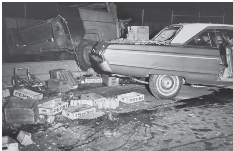
After this crash on the Gold Star on Nov. 29, 1967, in which three people were seriously injured and traffic was tied up for hours, letter writers demanded action from state officials and urged a higher median divider on the bridge. CONNECTICUT STATE LIBRARY
